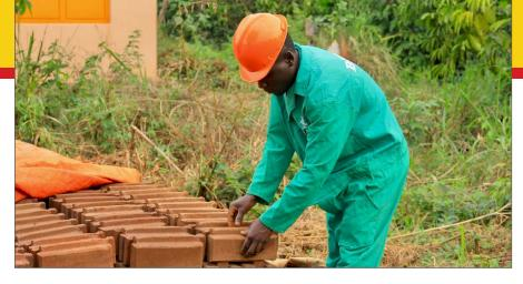
on big trucks. Because they are notched like a Lego, the builders need 83% less mortar in the layer between the bricks. And the finished walls look really sharp without needing to be plastered.
